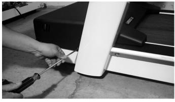
Attach motor cover with Phillips head screws provided. Plug treadmill into a dedicated 15A outlet.
